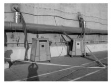
Fig. 7 picture of two ozone generators in action at a treatment of a large elevator Treating an entire structure is difficult; an alternative is to focus on the outlet silo semi continuous treatment.
